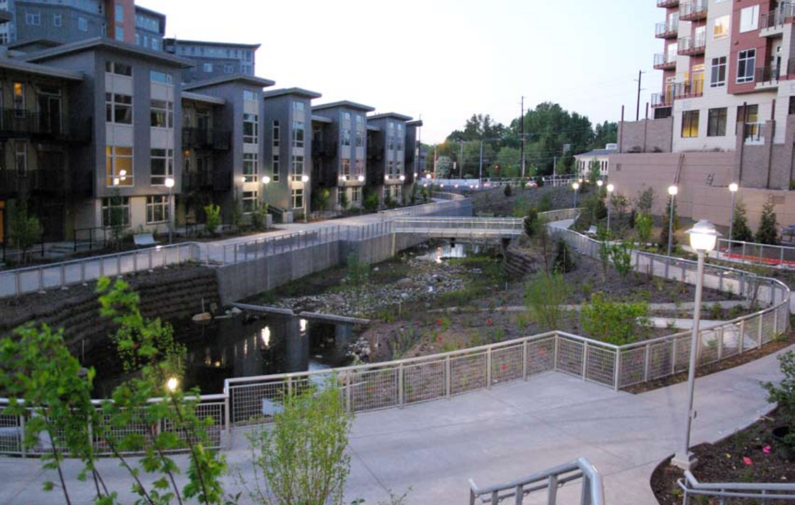
Thornton Creek Water Quality Channel at Night
